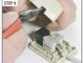
Notch the cover to match the cable entry and snap it in place.
