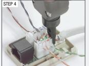
Insert the pairs to the color coded slots taking care to maintain the conductor twist at the IDC terminal. Punch down using a 110 style tool.
