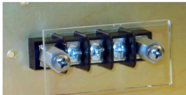
Installed Terminal Block
