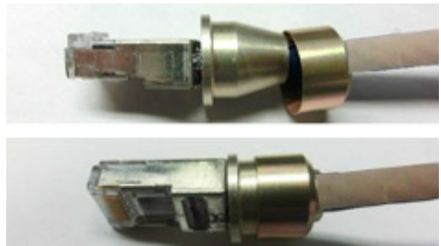
9.19 Bring the inner wedge up towards the RJ-45 and slide the outer wedge up to mate with the inner wedge.
